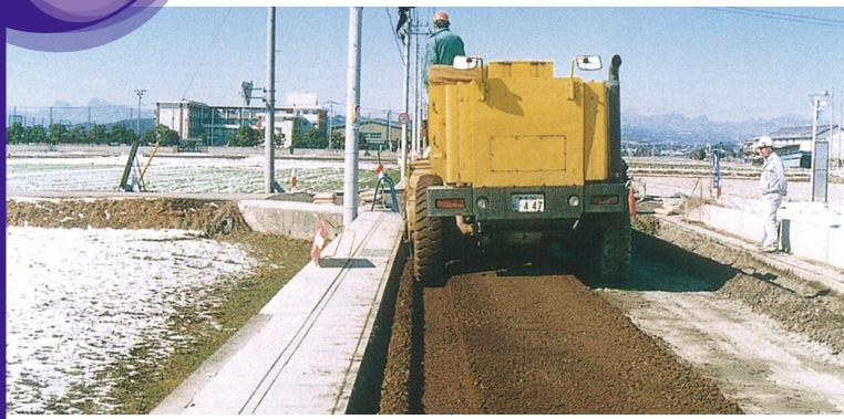
The existing asphalt mixture and subbase are crushed while on the road, and used as raw material for creating a new subbase.
